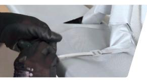
Secure the bandage with metal straps against slipping. Use at least two straps per bandage strip.
