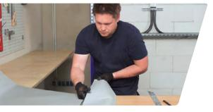
Measure the cable support system and cut the bandage to fit support areas. Allow for the bandage overlapping by  $\geq$  50 mm in longitudinal and transverse directions.
