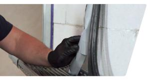
Wrap the bandage around protruding cables.
