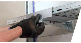
Wrap the bandage strips with the coated side facing inwards around the support system in the supported areas and restrain them temporarily with duct tape.
