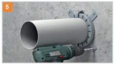
The pipe collars must be mounted to the rigid walls or floors through the fastening clip with appropriate dowels and steel screws M6 or M8.
