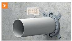
Finally apply the identification sign to the penetration seal. The identification must be place next to the penetration seal to the building component and is available at Kuhn.
