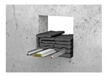
4. In floors with a thickness < 250 mm, non-combustible panels must be installed to reach the required minimum thickness of 250 mm. The fire protection pillows are held in place by a steel grid installed below the floor (≤ 40 × 40 × 4,8 mm, not included in delivery), onto which a glass fibre mat (≥ 125 g/m²) is placed.</p>
