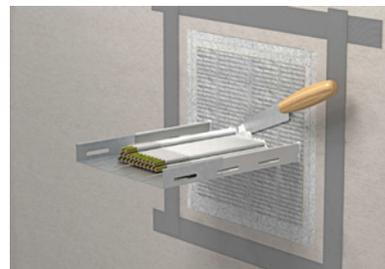
5. Coat the seal surface. Finally coat a 20 mm wide area around the installations with BML.
