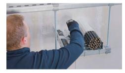
Finishing coat: Coat each side of the cable over a length of 100 mm in front of the penetration seal and the penetration seal surface, as well as an an extra length of 20 mm with BML.
