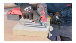
Take measurements for cutting the board to size, mark cutting lines and cut the board as required; make cutouts for the feed-throughs and check proper fit.
