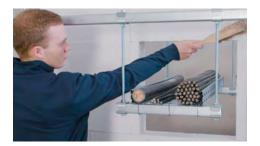
Clean the reveal surfaces of the component opening as well as the installations penetrants and mask the reveal with adhesive tape.
