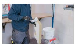
Stir the coating compound and coat the cables in the penetration seal area with BML; coat the component reveals and the edges of the mineral fibre board with BML or BMS/ BMK. Insert one or two boards into the opening.
