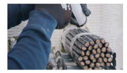
Stuff the remaining openings with mineral wool and fill with BMS/BMK.
